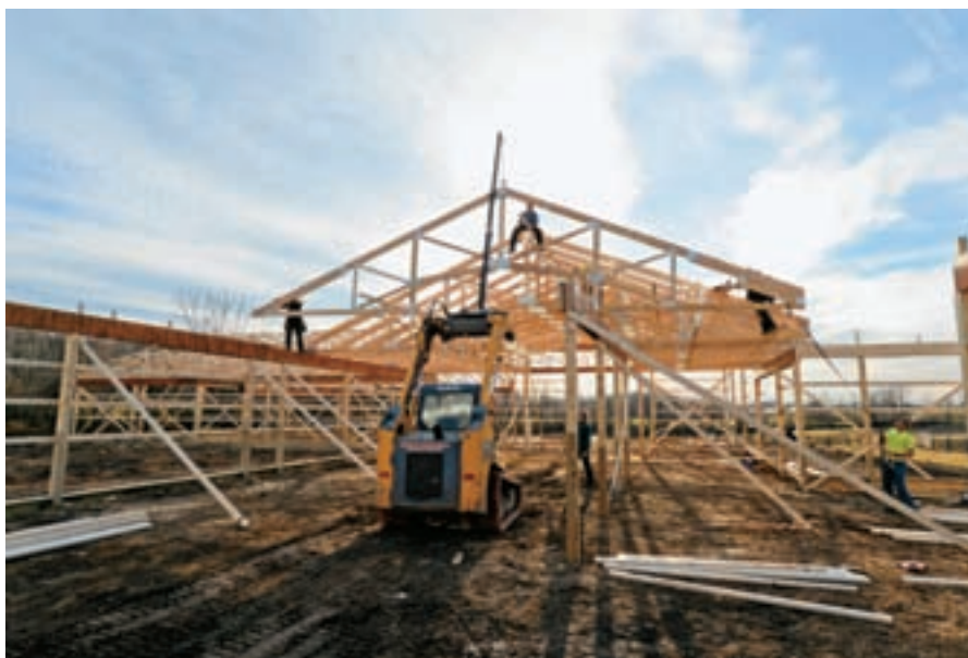
Construction on the new stallion barn at Saratoga Stud
