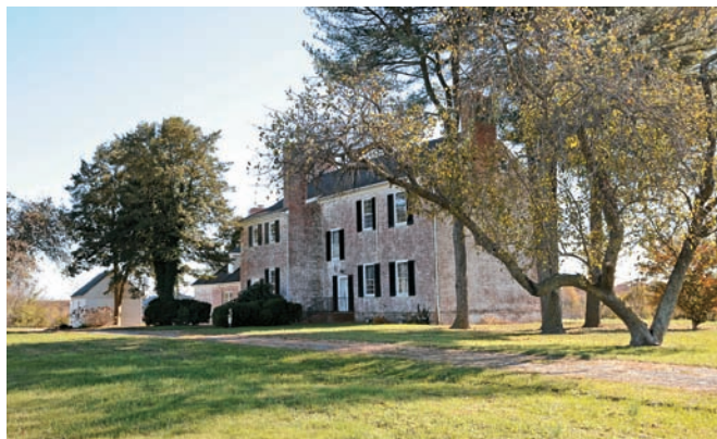
The main residence at Thornmar
