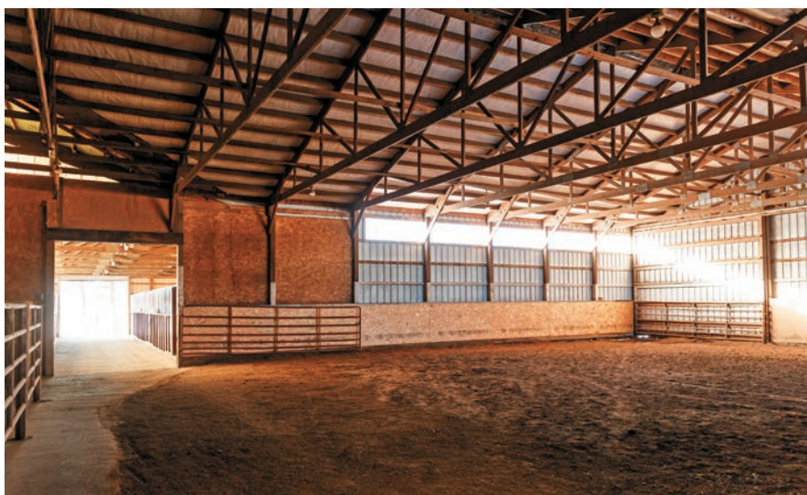
Solar-powered barn has a roof at a sharp angle, allowing the barn to capture sunlight in winter that can make the area 30-40 degrees warmer than the outside temperature
