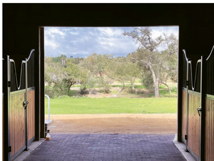
A renovated eight-stall barn on the property gives the farm flexibility as stalls have removable panels to convert the space into larger foaling stalls
