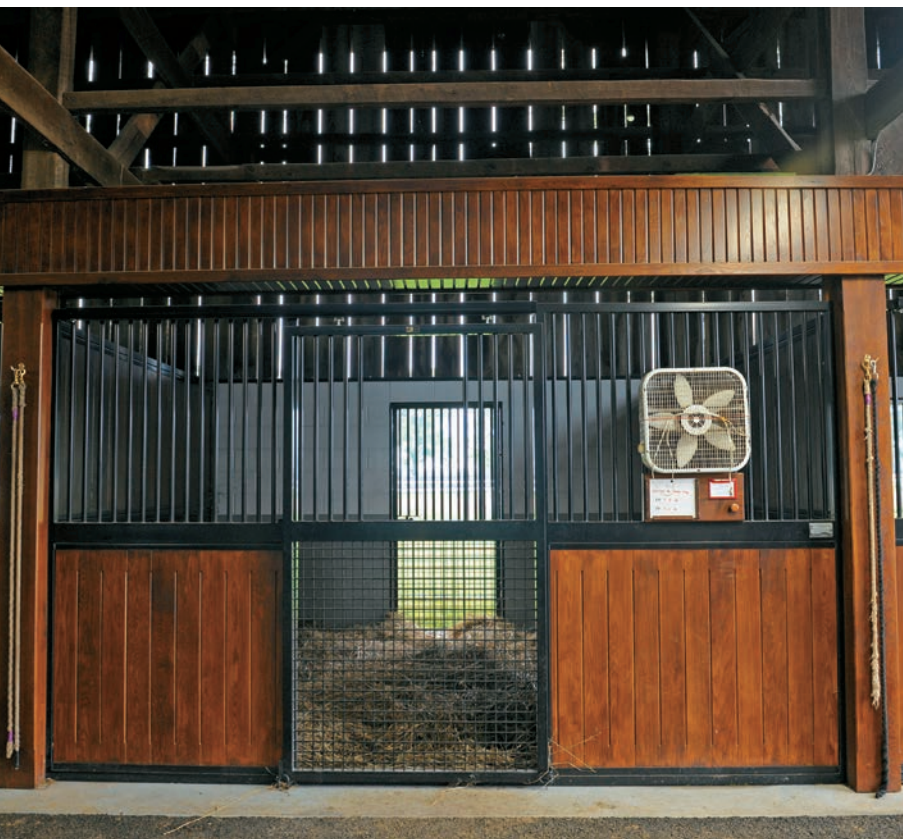
A barn at Margaux Stud near Midway, Ky. features front and back stall doors, which can speed up equine evacuation during an emergency
