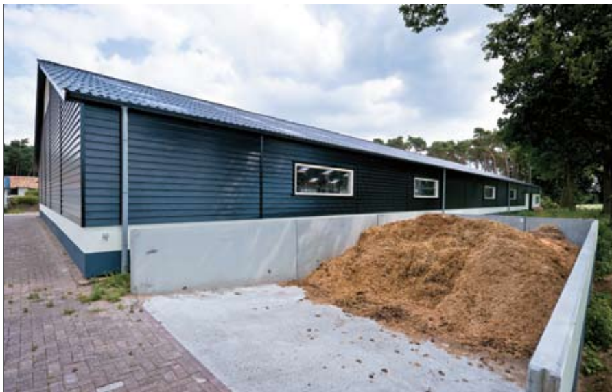
Using concrete bins for composting that allow the pile to be turned and managed with machinery makes the composting of horse manure a much easier job.
